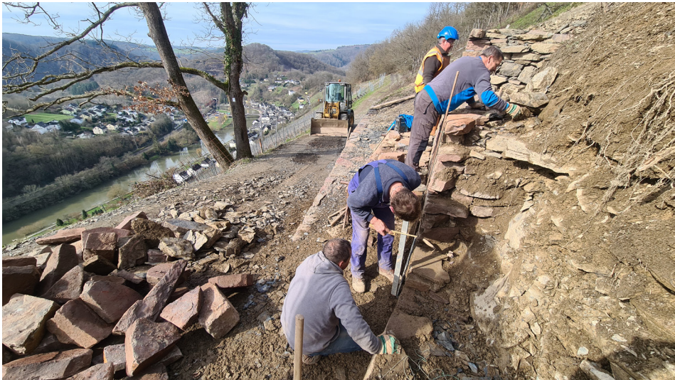
Figure 10. Work on a nature conservation wall by the VTG
